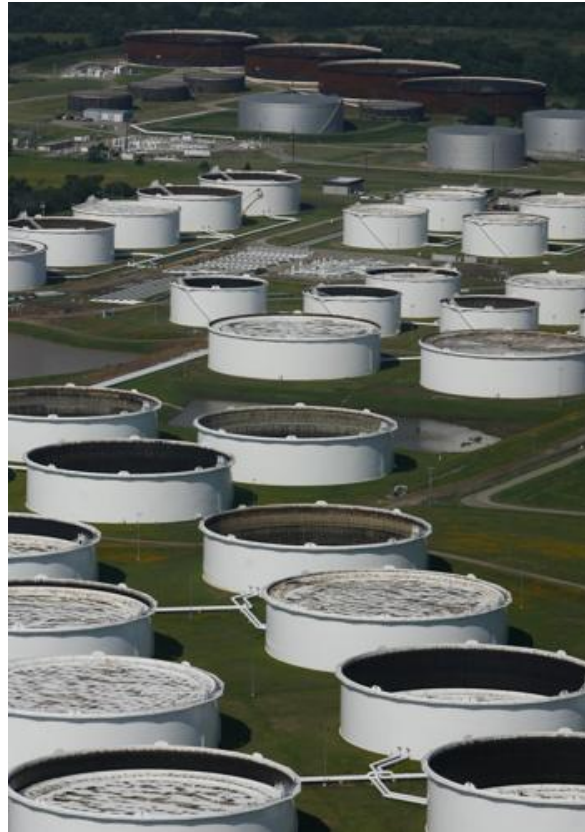
Petroleum storage tanks are shown in Cushing. Since the early 20th century, Cushing has been one of the world's leading pipeline junctions. Tulsa World File
